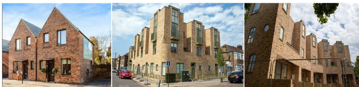
Council's Bury Street West, Maldon Road, Gatward Green developments completed in 2022/23
