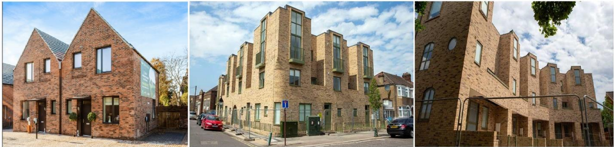
Council's Bury Street West, Maldon Road, Gatward Green developments completed in 2022/23
